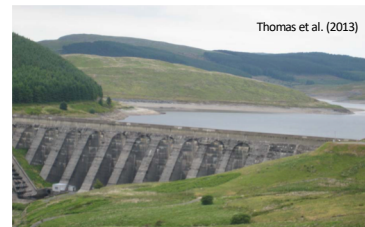
Figure 1.2. The Nant-y-Moch Dam in 2011 – No Symptoms of ASR after 50 Years – Constructed with Reactive Aggregate and 25% Fly Ash
