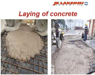
Fig. 6. Self-compacting concrete with LC 3
