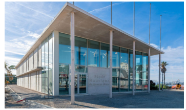
Stade Nautique du Roucas Blanc for 2024 Paris Olympic Games, Marseille, France. ECOPlanet concrete with a 40% lower CO 2 footprint made from calcined clay-based ECOPlanet cement
