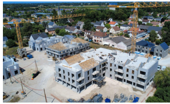
Le Clos Saint-Joseph residential development, Orléans, France Calcined clay-based ECOPlanet cement with a 36% CO 2 reduction used for precast concrete
