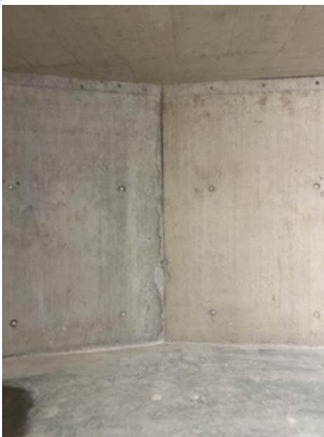
Conventional cement (left) and LC 3 (right) wall – Swiss example
