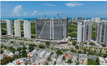
Woha Tower, Cancun, Mexico ECOPlanet with calcined-clay based cement achieving a 30% CO 2 reduction
